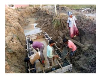
Photo 2.33: Reinforced concrete pouring for constructed wetland basement
