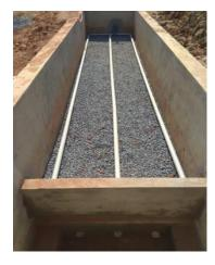
Photo 2.37: Gravel bed and pipeline work in constructed wetland
