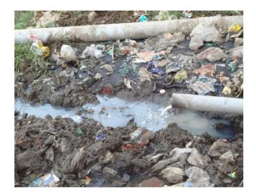
Photo-2.2: Wastewater being let out into open
