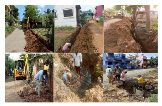
Photo 3.36: Pipe Laying Work in Phase -II Villages
