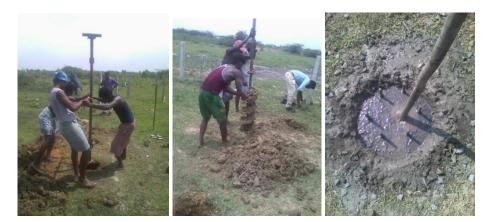
Photo 2.19: Pile Foundation Work: (15<sup>th</sup> July to 25<sup>th</sup> July)
