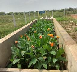
Photo 2.40: Waste water flowing vertically in the constructed wetland
