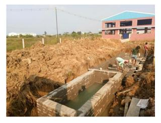
Photo 2.34: Fly ash brick work for constructed wetland
