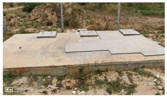
Photo 3.12: Photograph of three chambered septic tank (60 m<sup>3</sup> capacity)
