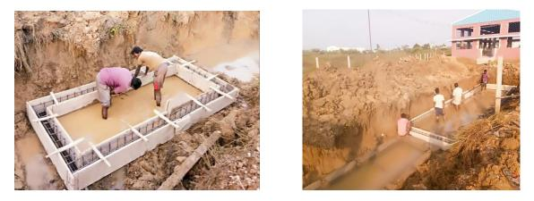
Photo 2.32: Shuttering and steel reinforcement for constructed wetland basement
