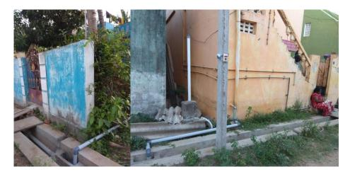
Photo 2.31: Households connected their grey water into main sewer water pipeline
