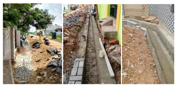
Photo 2.26: Civil work- Storm water drain constructions near households
