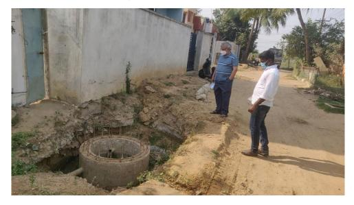
Photo 3.37: Flow test monitored by IITM team to ensure gravity flow of wastewater
