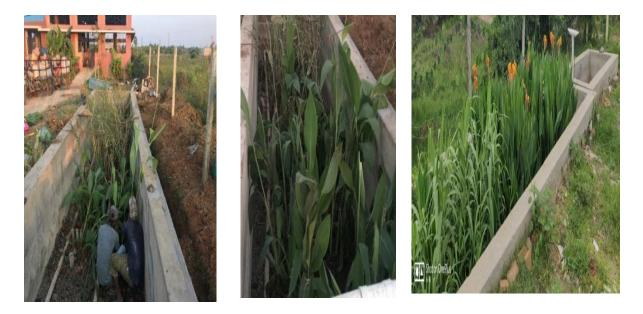
Photo 3.18: Photographs taken during and after re-plantation of plant species in constructed wetland
