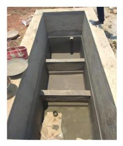
Photo 2.35: Construction of settling tank
