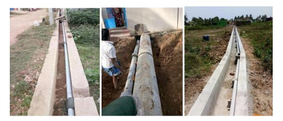
Photo-2.30: Civil work: Sewer water pipeline constructions
