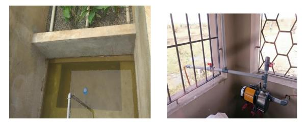
Photo 2.42: Treated water from constructed wetland is pumped into overhead tank for reuse (for compost preparation and washing)
