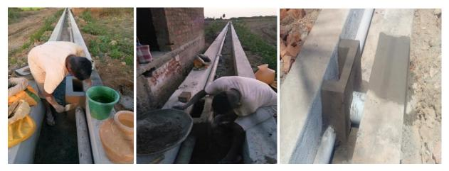
Photo 2.28: Civil work- Construction of sewer water pipeline and chambers
