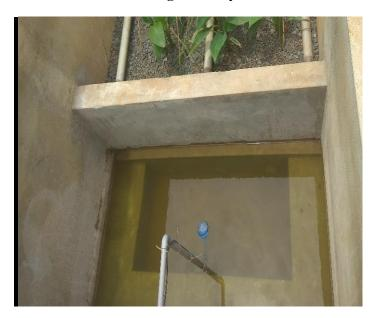
Photo 2.41: Treated water coming out to the outlet chamber
