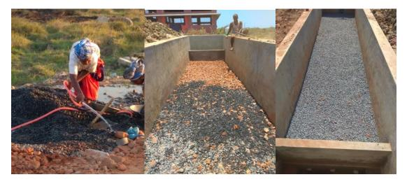
Photo 2.36: Formation of substrate (Gravel and bricks) bed for constructed wetland
