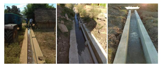
Photo 2.29: Water Flow Test on Storm water Drain
