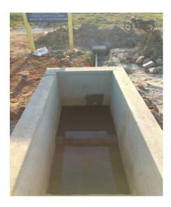
Photo 2.39: Waste water coming into settling tank
