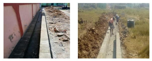
Photo 2.27: Civil work- Storm water drain constructions near open land
