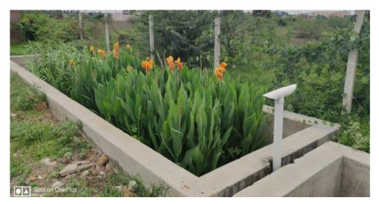
Photo 3.11: Vertical flow constructed wetland with two varieties of plant species namely Canna indica and Phragmites australis
