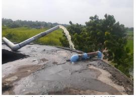
Borewell supply- Discharge at roof level of OHT
