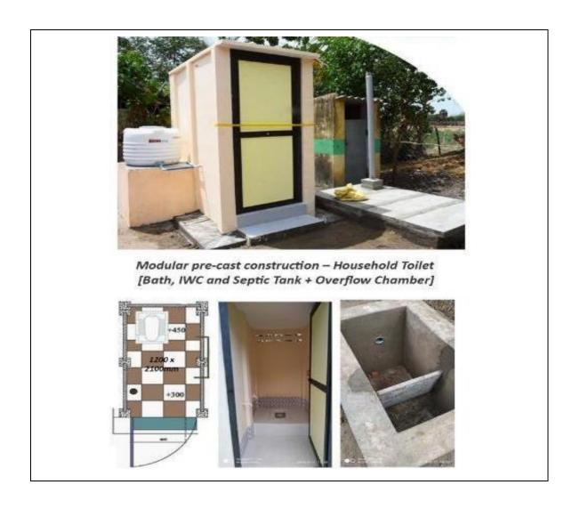
**4.2.3 Septic Tank Construction Design:** The design of Two compartment Septic Tank with overflow chamber arrangement is shown below:
