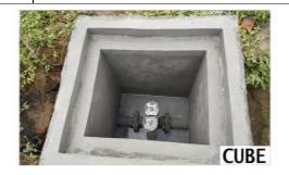
Valve chambers and Gate valve fixing under progress
