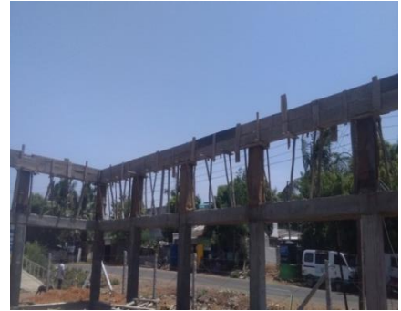
Fig. 22. RCC for Second Lintel Beam: 7-7-2018
