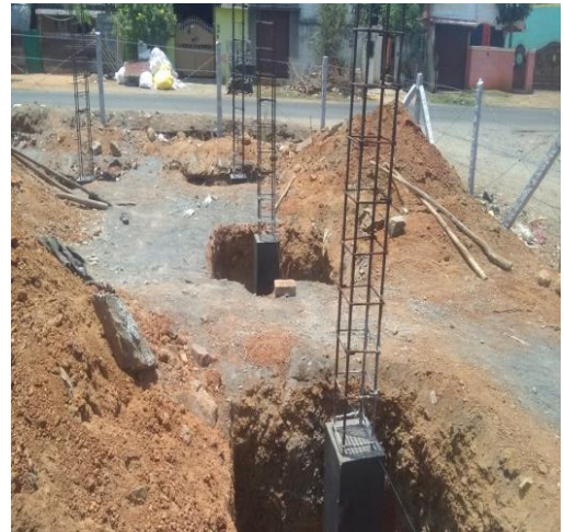
Fig. 16. Reinforcement of Footings: 14-05-2018
