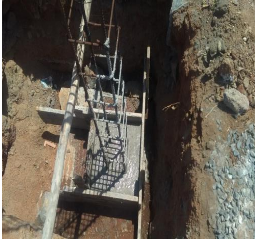
Fig. 16. Reinforcement of Footings: 14-05-2018
