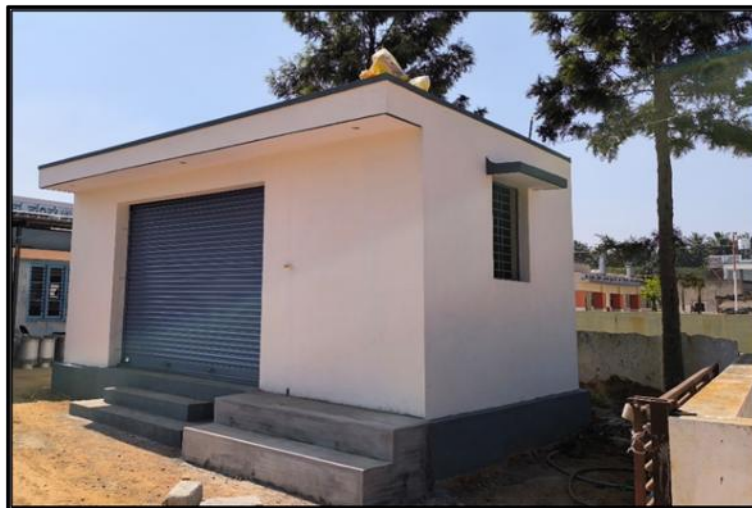
Fig.4. WTP at Ankathatti Dairy Farm
