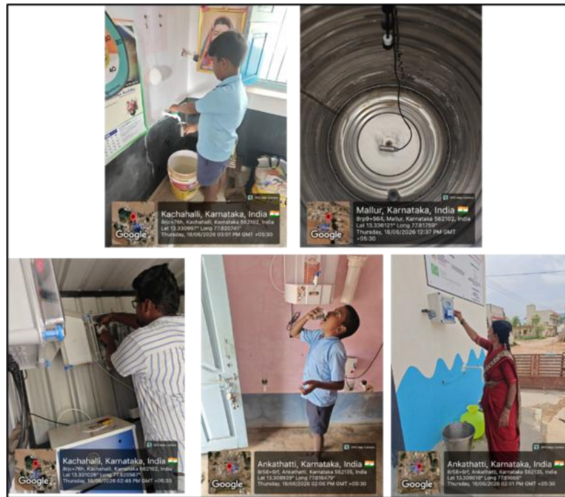
Fig. 6: Drinking Water Treatment Systems in Mallur Panchayat
