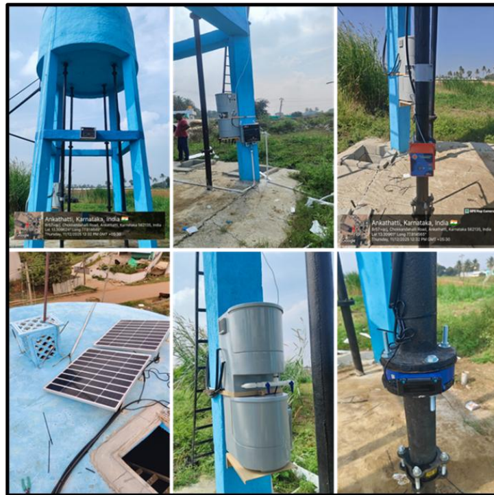
Fig. 7: Electrochlorinator Installation
