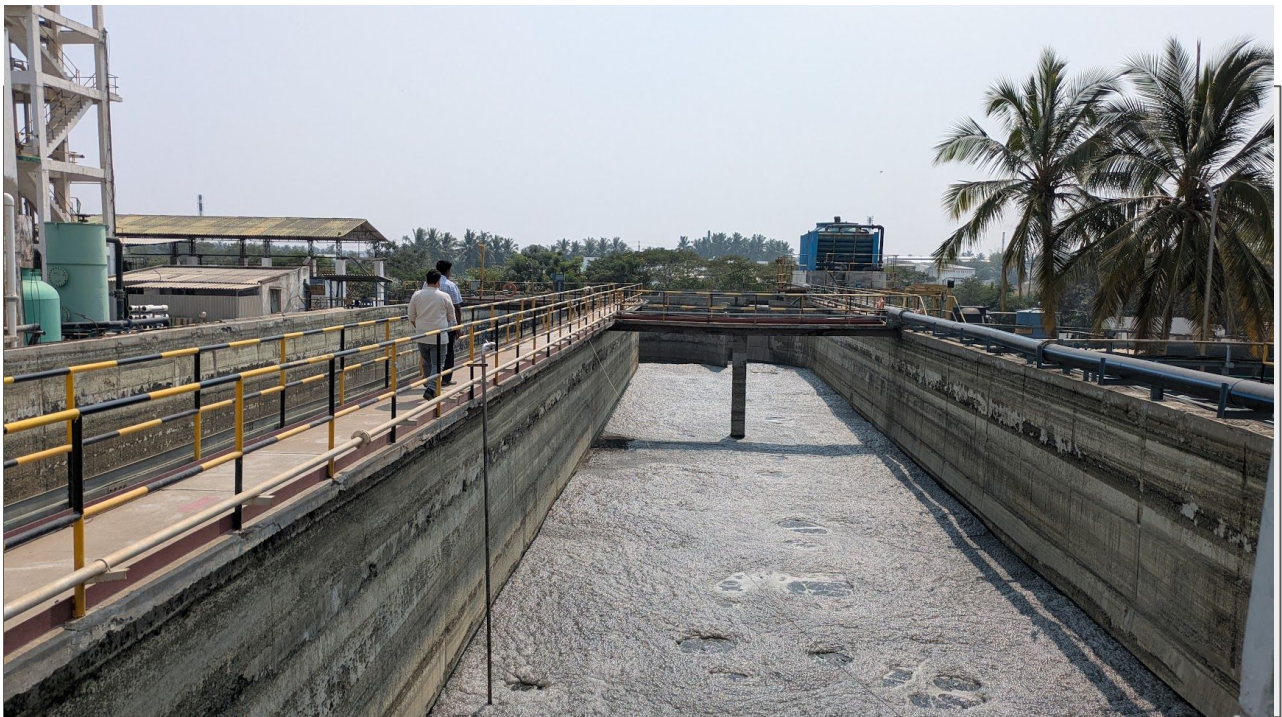
Figure 5.0: A visit to the sewage treatment plant at Tiruppur. Source: WELL Labs, 2026
