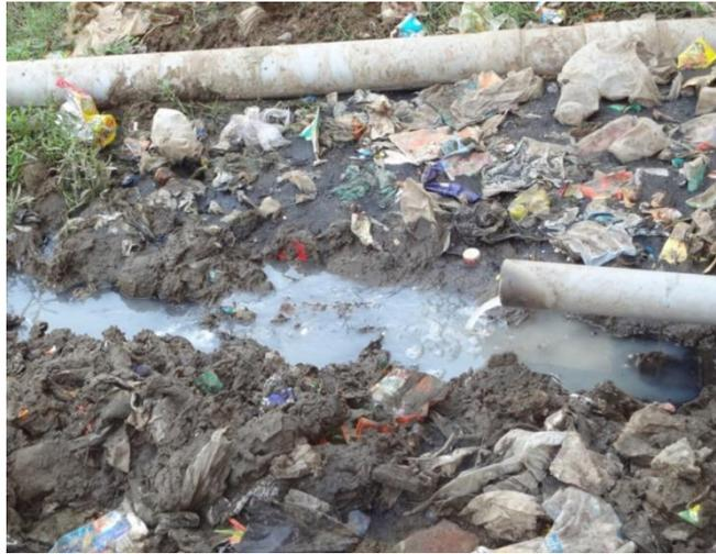
**Photo-2.2: Wastewater being let out into open**
