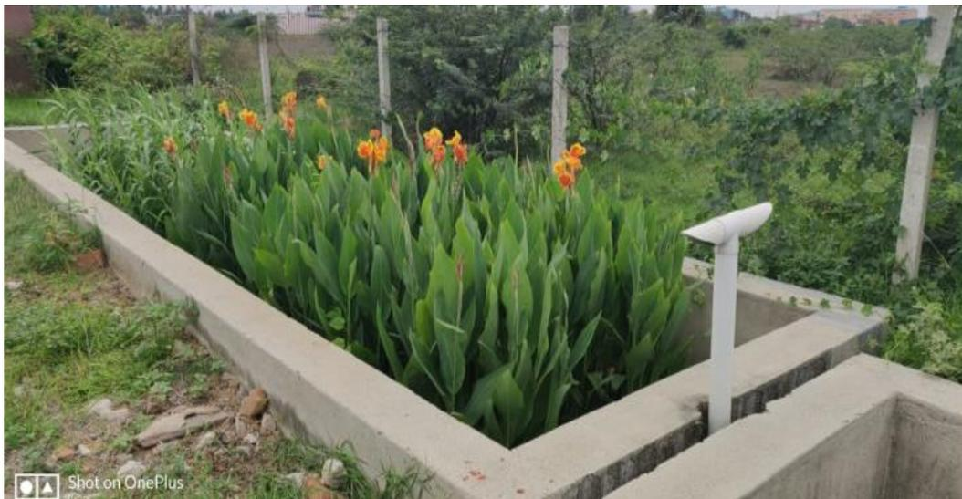
**Photo 3.11: Vertical flow constructed wetland with two varieties of plant species namely *Canna indica* and *Phragmites australis***
