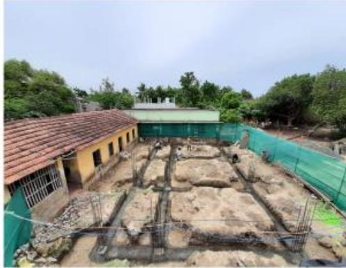
Footing RCC Completed & Grade Beam in Progress
