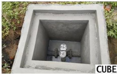
Valve chambers and Gate valve fixing under progress
