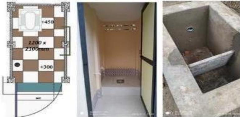
**4.2.3 Septic Tank Construction Design:** The design of Two compartment Septic Tank with overflow chamber arrangement is shown below:
