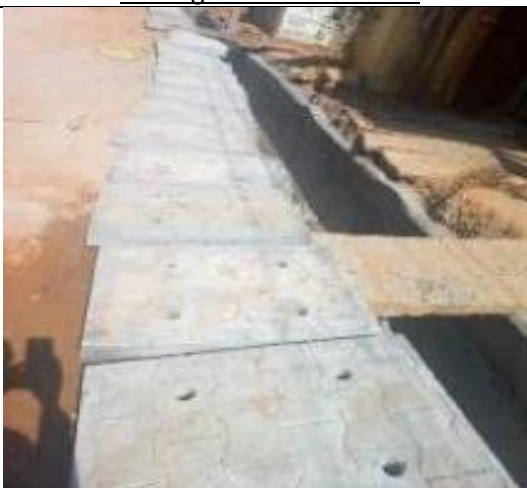
Placing of Precast slabs
