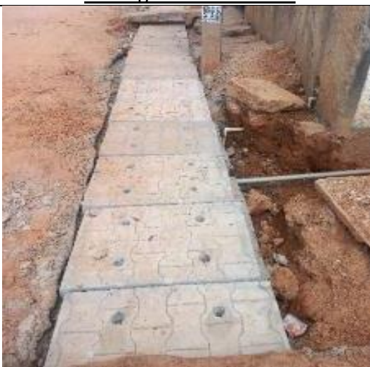
Placing of Precast Slabs
