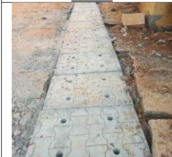
Placing of Precast Slabs
