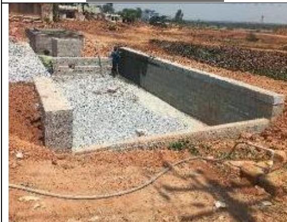
Laying of 20 mm Gravel (Bottom Layer)
