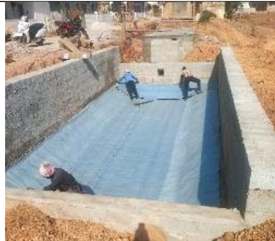
Laying of Geomembrane
