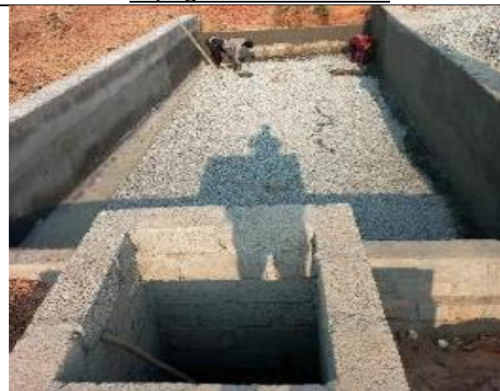
Laying of 20 mm Gravel (Bottom Layer)
