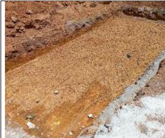
Excavation for wetland
