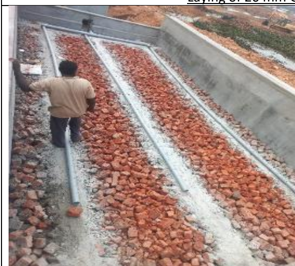
Laying of Brick bats
