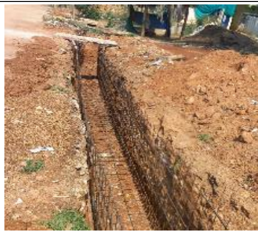
Placing of Reinforcement
