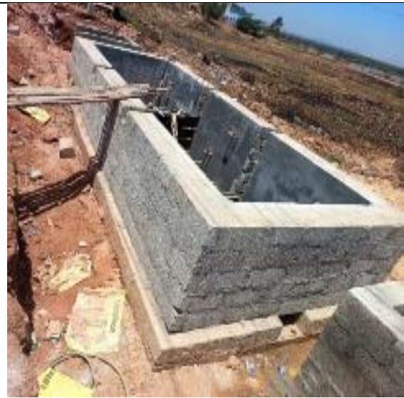
Completion of Blockwork
