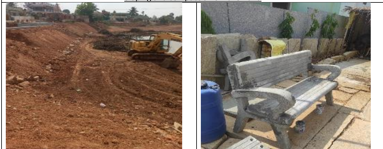
Sloping of Lake Bund
