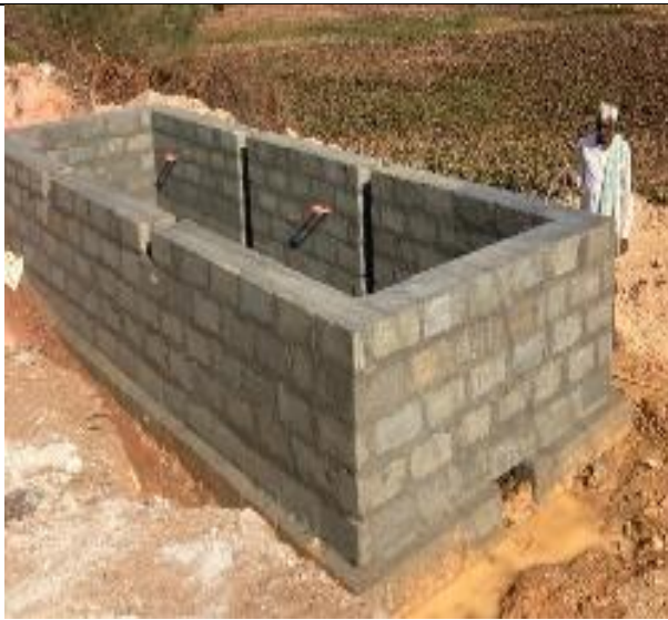
Completion of Blockwork
