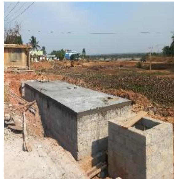
Casting of Slab
