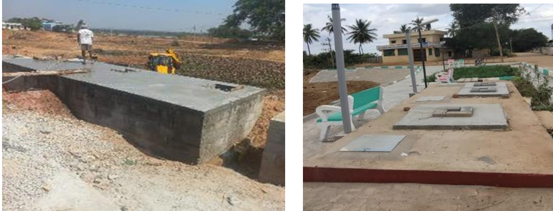
Fig.8: Construction of Septic tank
