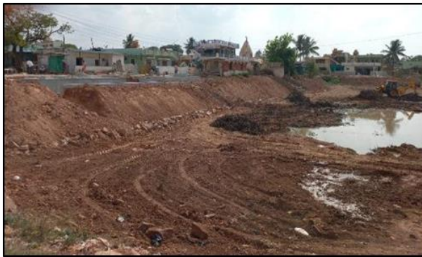
Fig. 12: Lake bund repairs
