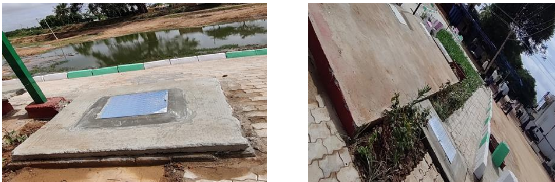
Fig.9: Inspection Chambers
