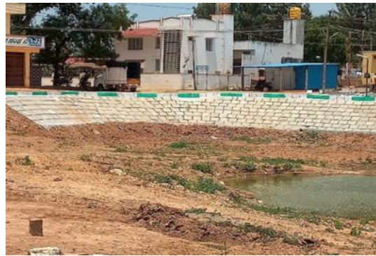
Fig. 12: Lake bund repairs
